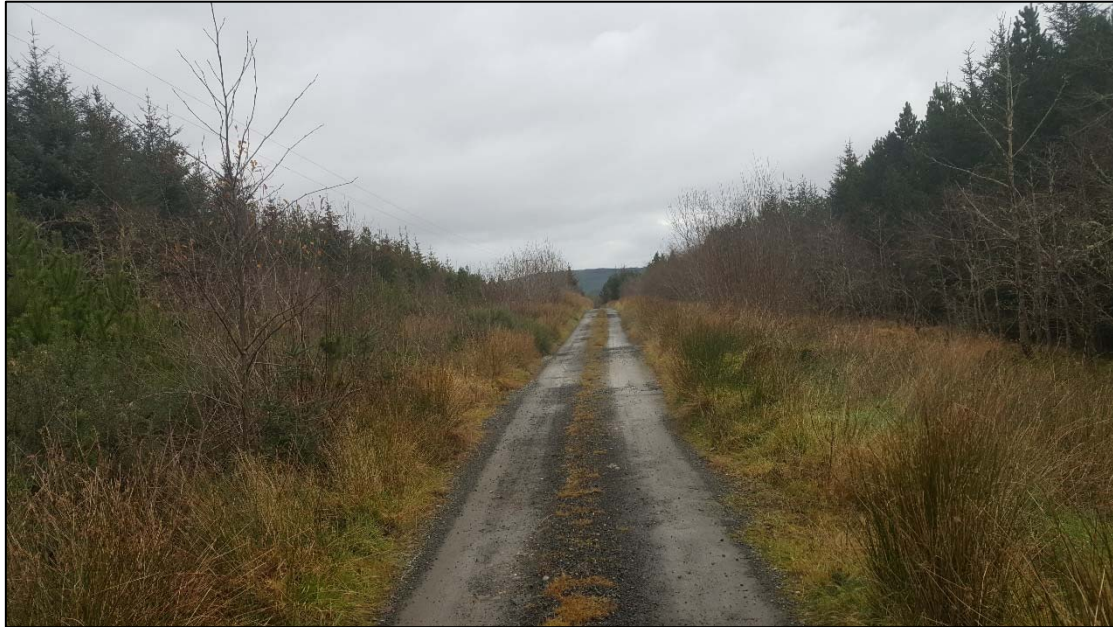
Plate 6-15 Local public road in the townland of Meenyanly along which the proposed cable route will be located.
