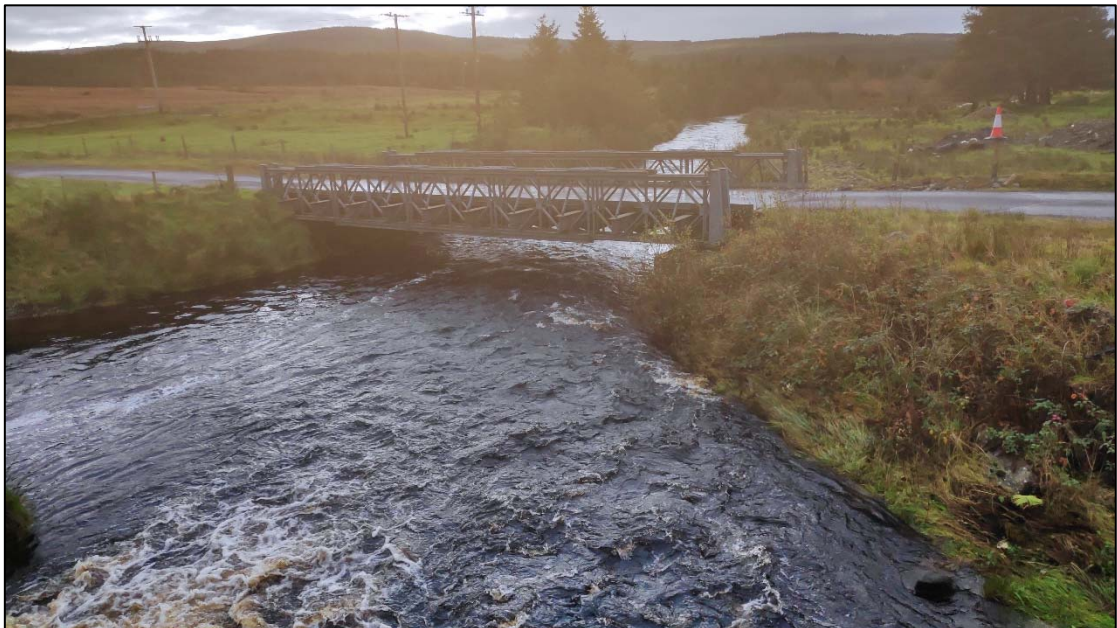
Plate 6-7: Eroding/upland river (FW1), the Crana River, located to the north of the EIAR study area boundary.
