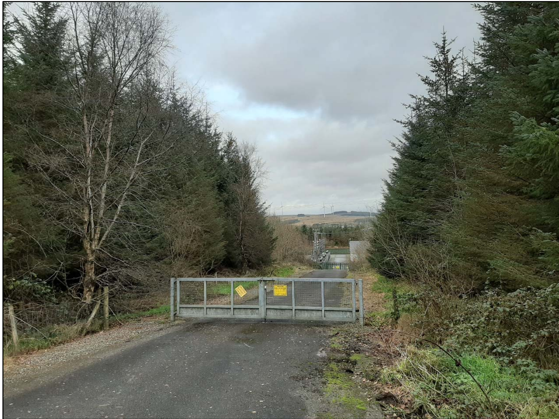
Plate 6-18 Access track to the existing Trillick substation and adjoining forestry (WD4).
