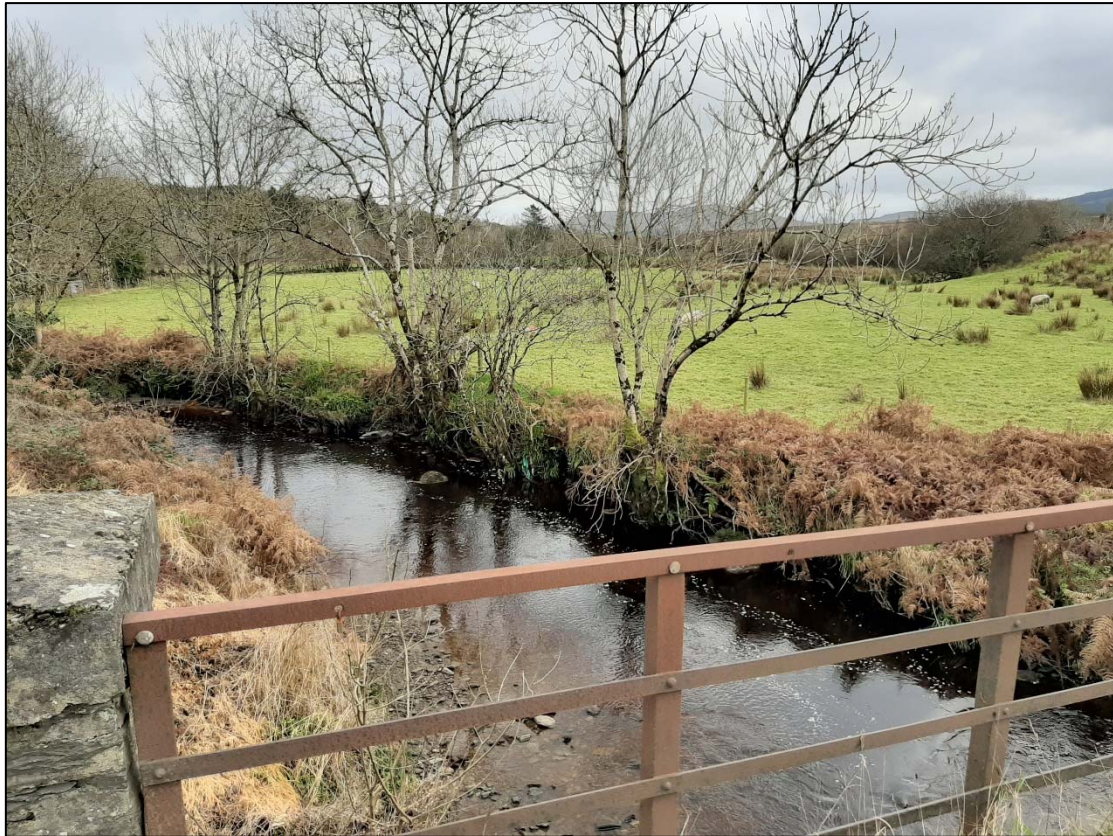
Plate 6-17 Bridge at Tullydish Upper, spanning the Owenkillew River, across which the proposed grid connection route will pass.
